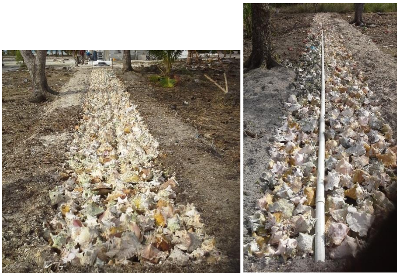
Figure A-6: Leach Field with Crushed Conch Shells at Little Water Caye (Photos taken by Christine Prouty)
