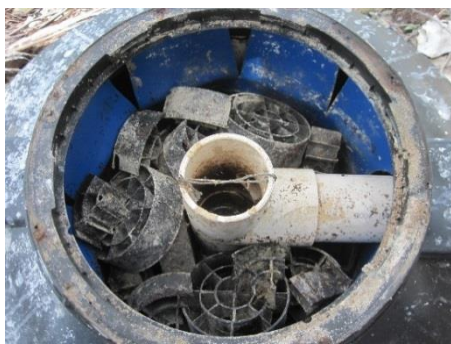
Figure A-9: Inside of Semi-Anaerobic Biodigester at Silk Caye (Photo taken by Christine Prouty)
